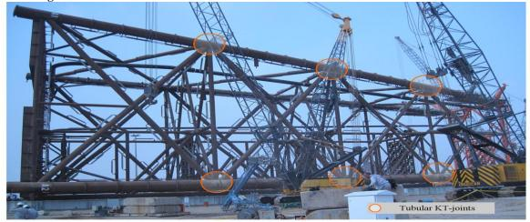
(a) Tubular KT-joints in a jacket structure during the fabrication
